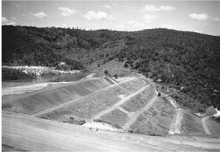
Figure 7. General view of Monjolo Dam (2000).
