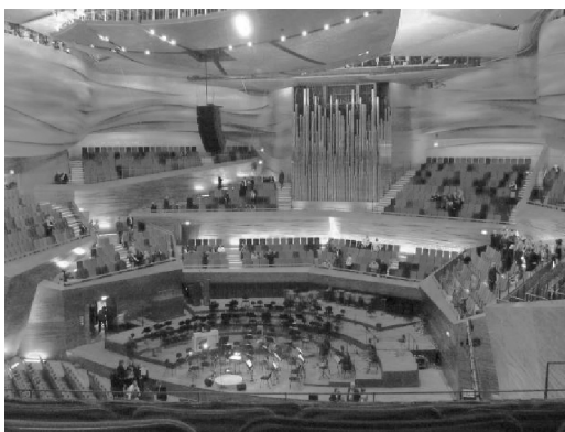
Figure 10. Curved risers and high canopy in the new Danish Radio Concert Hall in Copenhagen.
